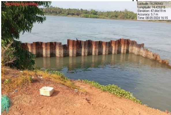
Approach Trestle 2 - Sheet Piles Driven and Liner Fabrication
